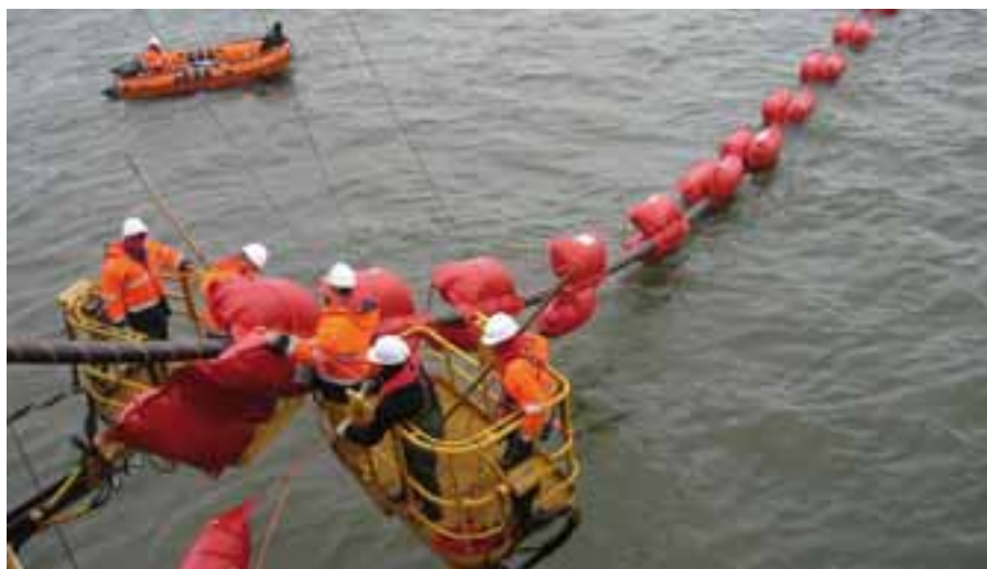
The NorNed high-voltage power cable is being laid in the North Sea.
