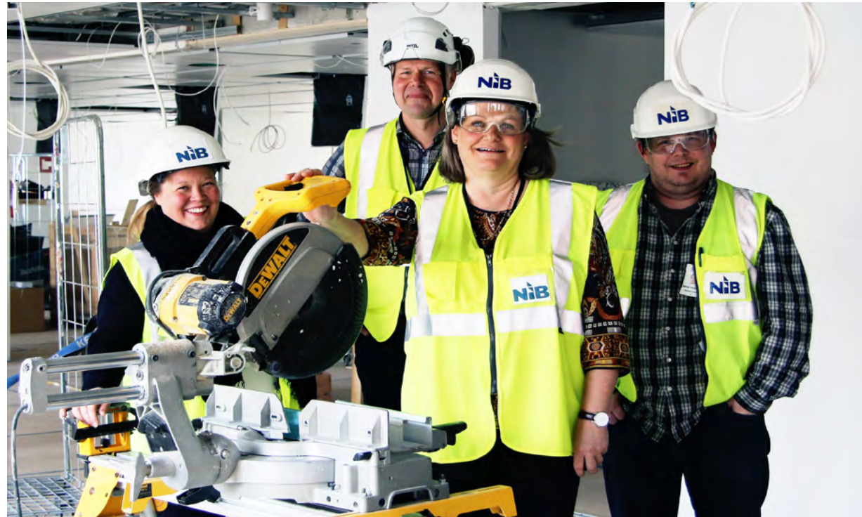
NIB's office renovation team. From left: Sophia Tuukkanen, Pasi Viitaniemi, Elina Mustonen and Mikael Söderbäck
